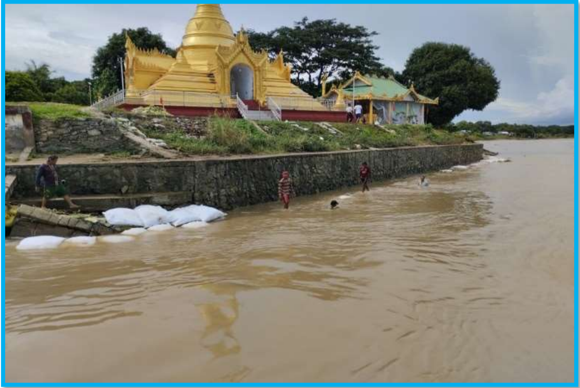
Condition Before Starting Work
