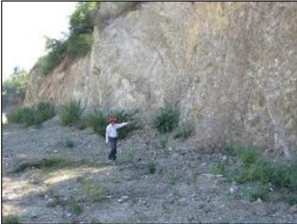
Figure (2) Rockfall at the western part of Yinmabin
