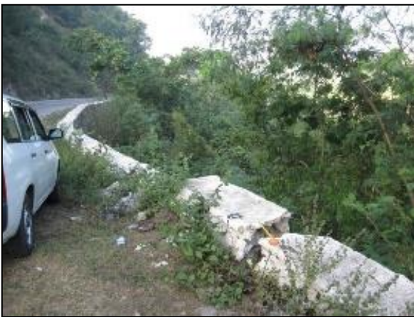
Figure (4) Creep by river bank erosion at the eastern part of Yinmabin
