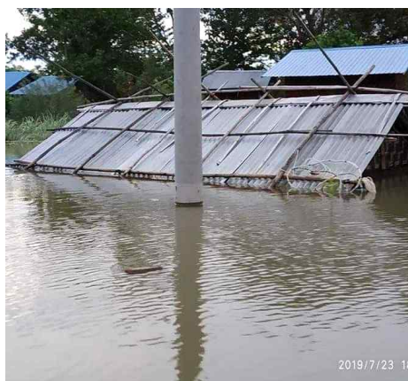
Image 2. Submerged homes in Kyauk Thawe Tauk village during flooding in August 2019 flooding in (Source: Photo taken during survey)
