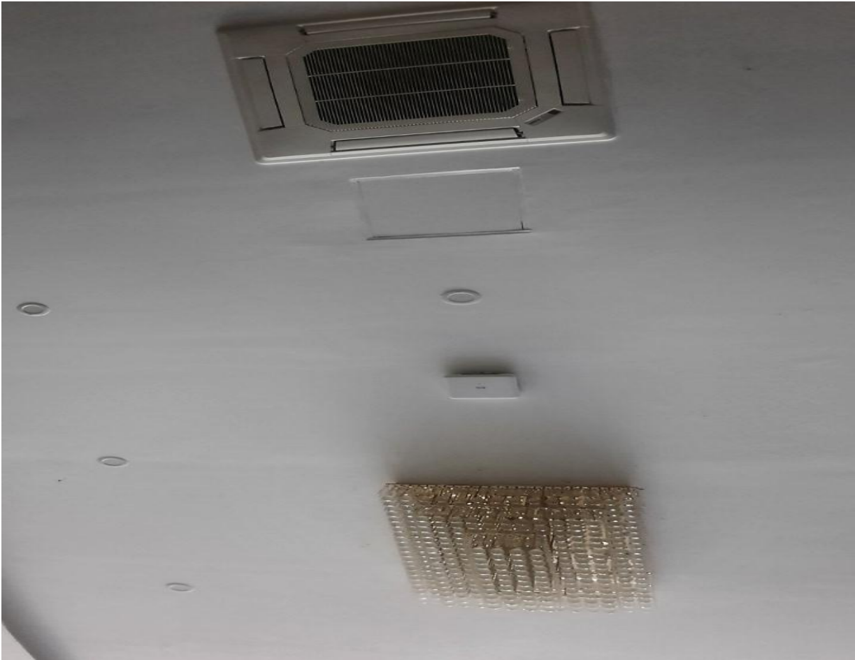
Wi-Fi Router set up on ceiling
