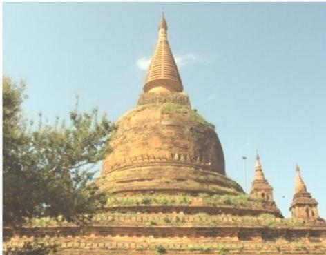
Fig-16, Hemispherical dome and square crowning block of the Setanagyi Stupa
