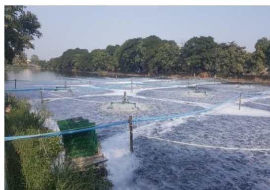
Figure 5. Surface Aerator on the water canal
