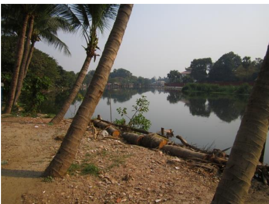
Figure 6. Finishing part of Thingazar Chaung
