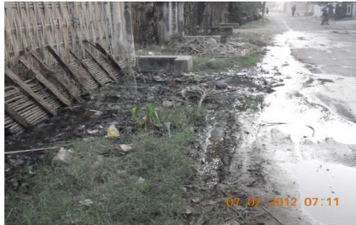
Photo(3) Flooding of gray water due to blockage of solid waste in road side channel
