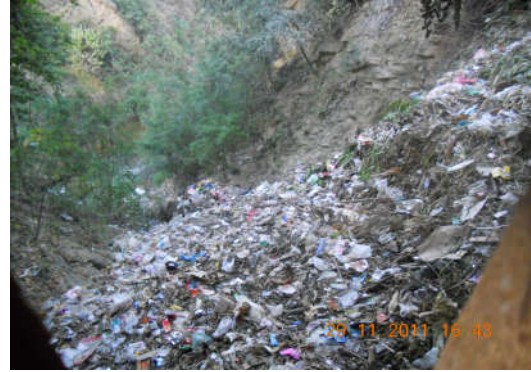
Photo(2) Disposing of Solid Waste into the Conduit from Meiktila Lake (N)
