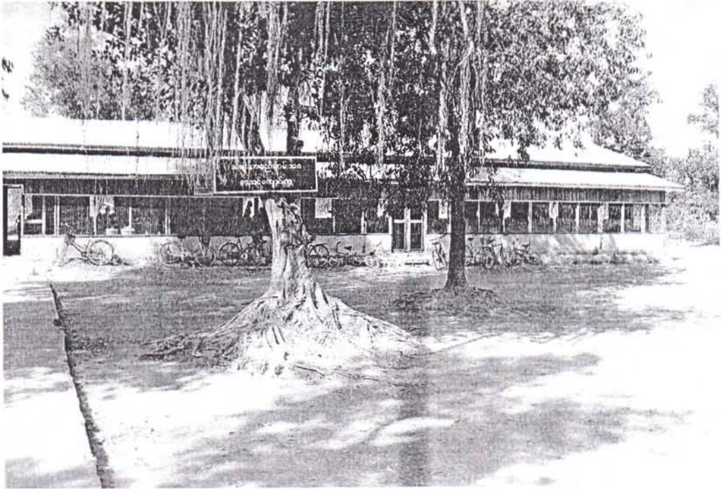
Main Building of School (Sitpinquin)
