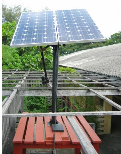
Figure 5. Photograph of solar panel tracking system
