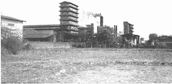
Fig. 10: One of the famous liquor factory in Shwepyitha Industrial City Part 1 which use boiler, fuel by paddy husk and pouring out the fume into the air as there is no control for it. (Photo: Zin Nwe Myint 2002)
