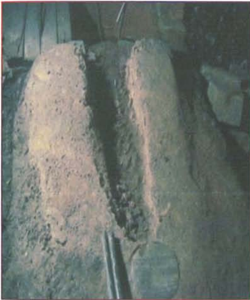
Figure-(4.35) Making the scaffolding
