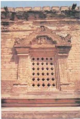
Figure 9. Perforated stone window of Nan-Hpava
