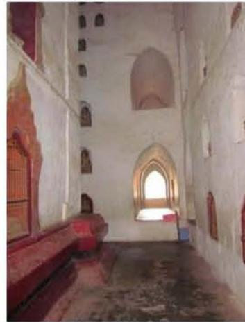
Figure 5. Double-layered windows through the wall to get light, Ananda
