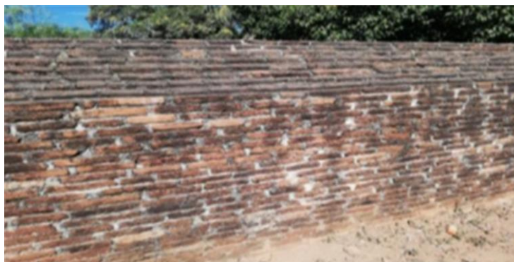
Figure 4 The wall between the Palace Hill and Shwe Yaung Taw Pagoda
