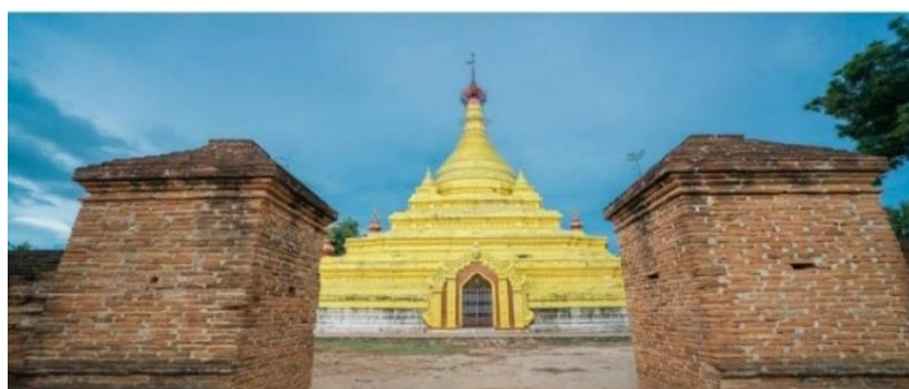
Figure 5 Two brick pillars of the Entrance
